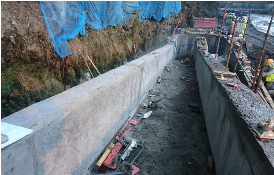
Upper sloping channel base and walls completed
