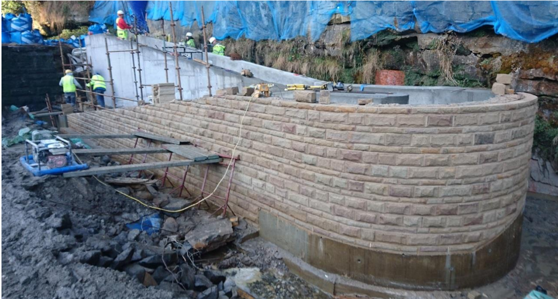
Masonry cladding completed to front wall, other than coping stones
